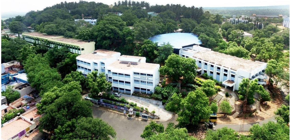
Fig. 9 Aerial View of JAC
